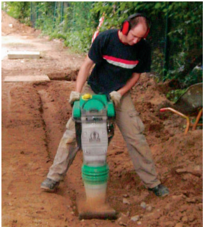
Abb. 3: Wacker-Vibrationsstamper BS 60-2
