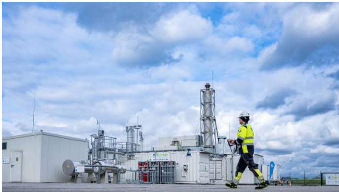
© Uniper Energy Storage
